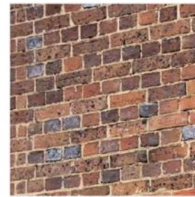
SOUTH BOUNDARY WALL EXPOSED RED BRICK (RE-USE HERITAGE REDS)
