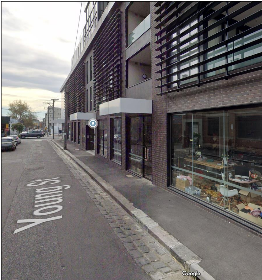
Figure 3 - Subject site (Tenancy 2 entrance) viewed from Young Street, looking toward Johnston Street - March 2020. Source: Google Streetview.
