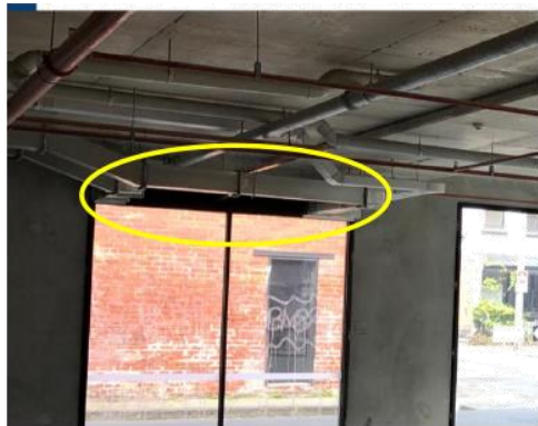
Figure 4: Ventilation louvres – internal view
