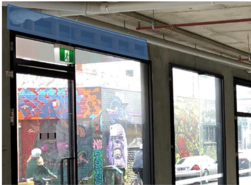
Figure 2: Opening above the glazing
