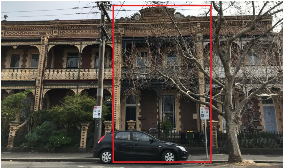
Figure 1: View of subject site from Gore Street (Planning Officer, August 2021)
