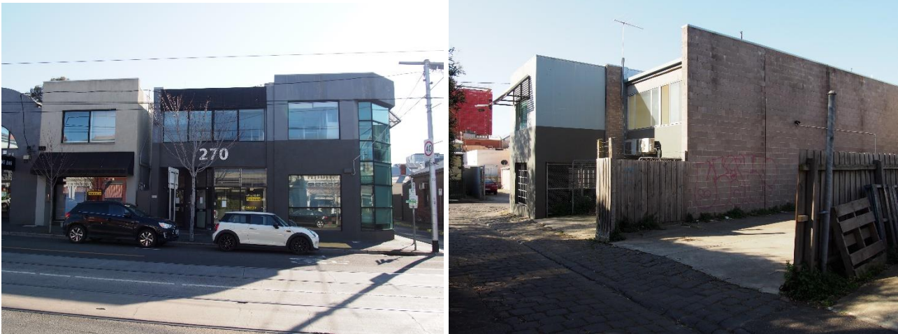
Photos: Subject site viewed from Church Street (left) and ROW (right)
