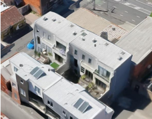
Figure 13: 3D Aerial images of No. 1/3 and 2/3 Little Oxford Street Source: Google Maps image capture date: 2021
