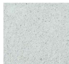
CON-01 OFF-FORM CONCRETE FINISH
