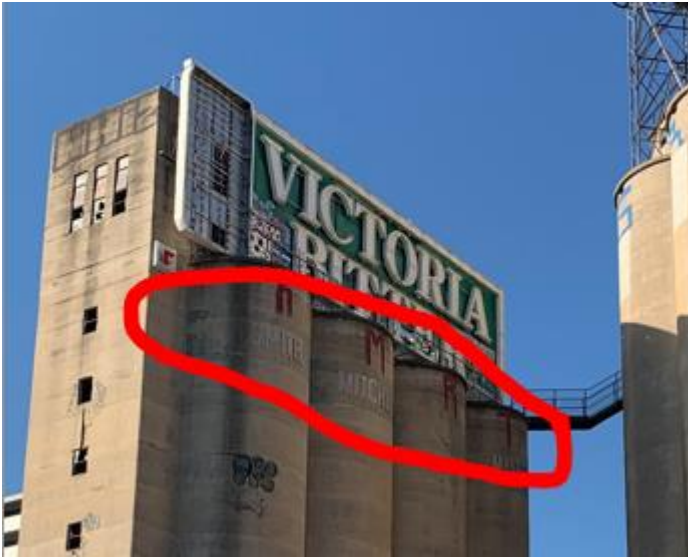
Figure 29 – existing silo building
