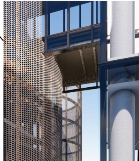
GLASS BRIDGE WITH STEEL BEAM STRUCTURE SLAB
