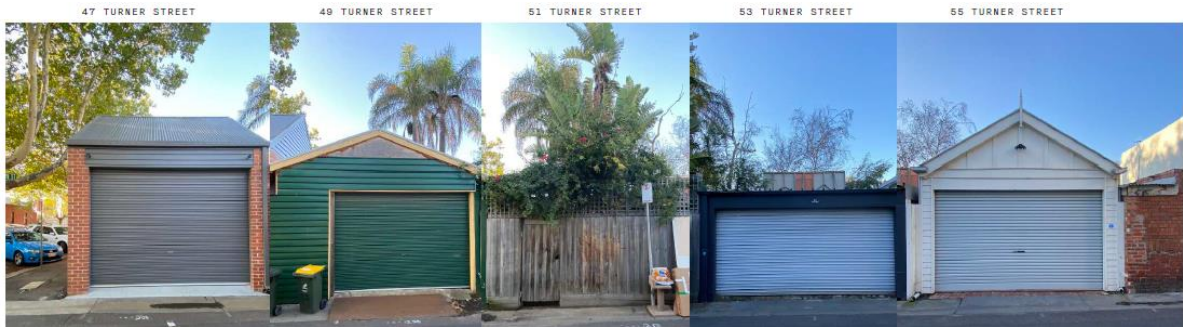
Figure 7: Garages of four out of five Turner Street dwellings facing Little Turner St. (Applicant submission, 2020)
