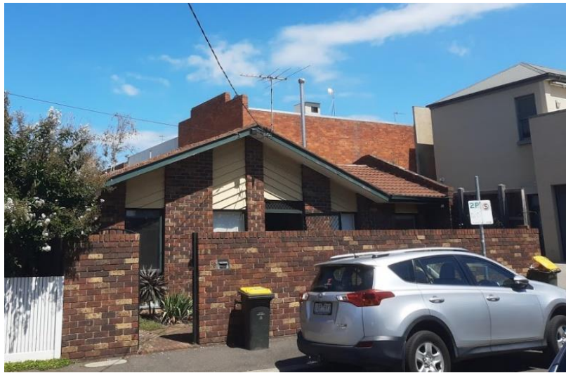
Figure 12: Dwelling to the north-east facing onto Farmer Street that has its rear to the laneway (photo taken 22/02/2021)
