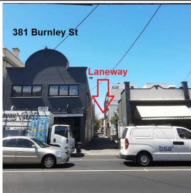
Figure 10: No. 381 Burnley Street and laneway viewed from Burnley Street (photo taken 22/02/2021)
