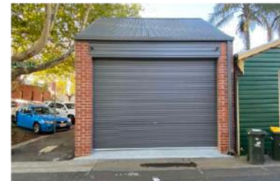
PHOTO - REAR OF 47 TURNER ST
