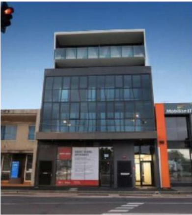
370 JOHNSTON ST 6 STOREY BUILT
