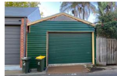
PHOTO - REAR OF 49 TURNER ST
