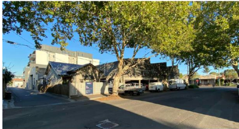
10. Rich Street facing South East toward Subject Site, 2 Rich St to the left and 350-356 Johnston Street to the right.
