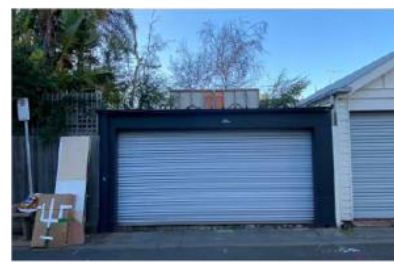
PHOTO - REAR OF 53 TURNER ST
