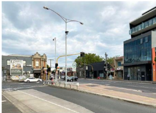
4. Johnston Street facing North West toward Rich Street. Existing facade.
