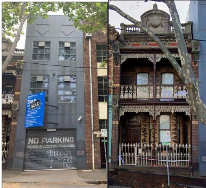
Figure 3 (left) Recent tilt-slab construction at 8 Peel Street, Collingwood. (right) Victorian Terrace at 6 Peel Street, Collingwood.
