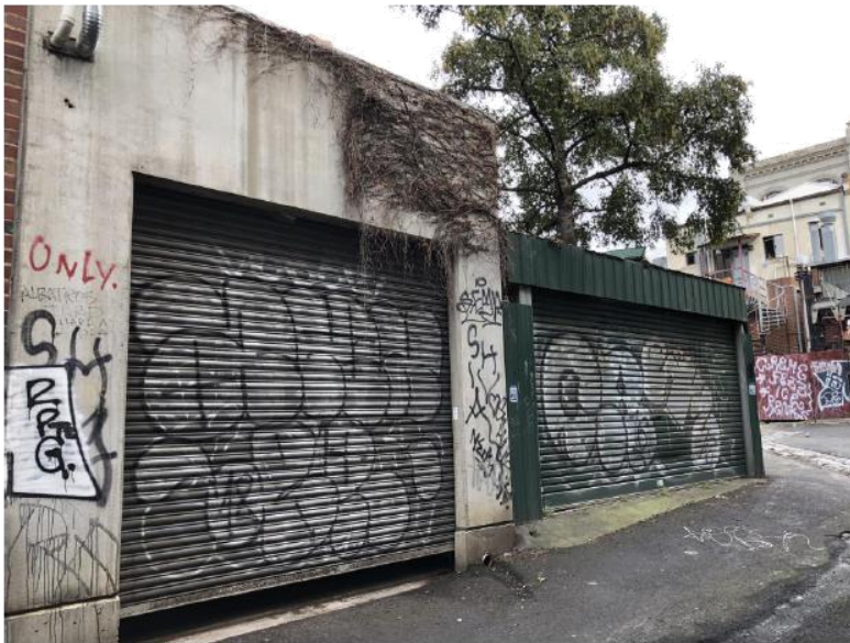
Figure 6 Rear (north side) of 8 and 6 Peel Street
