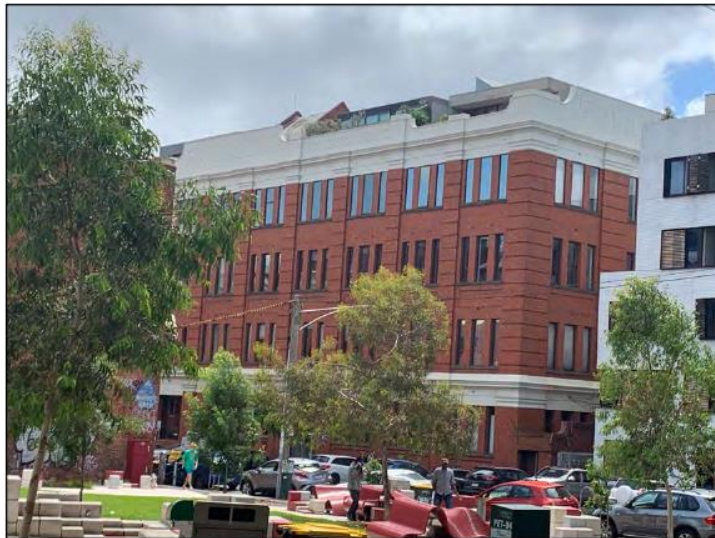
Figure 14 A former industrial building at 68 Oxford Street that has recently been repurposed for apartment living. Note the visible upper level addition set back behind the parapet.
