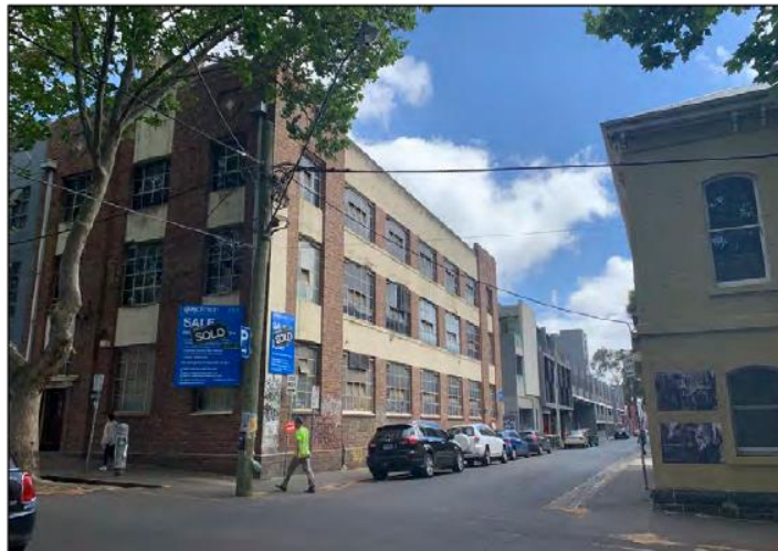
Figure 6 Looking north up the west side of Little Oxford Street.
