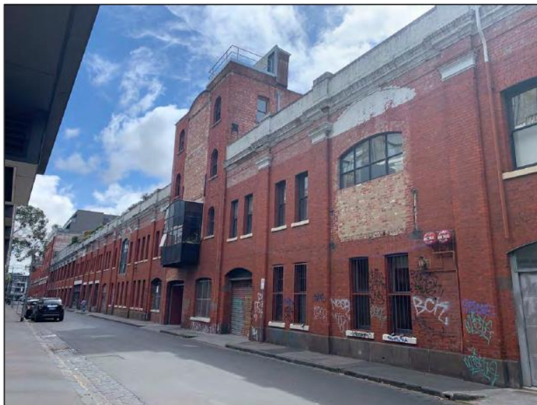
Figure 8 Red brick industrial building north the subject site, on the east side of Little Oxford Place.
