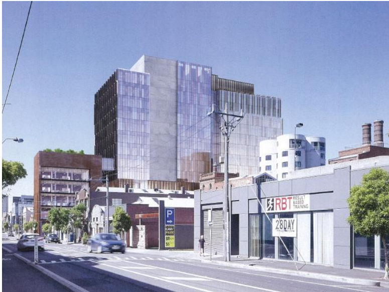
Figure 2: Photo montage of 2-16 Northumberland Street
