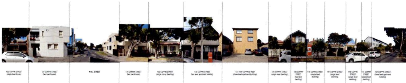
EXISTING STREETSCAPE - COPPIN STREET - EAST
