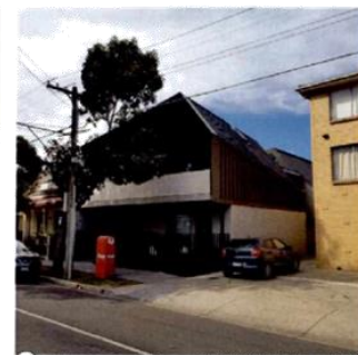
5 View from Coppin Street looking at two level development at 135 and 137 Coppin Street
