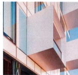
SUN SHADES AND DAYLIGHT SCOOPS projecting metal shrouds facing the park protect office interiors from the summer sun whilst allowing winter sun deep into the plan, with the angled base helping to reflect additional winter sun into the interior
