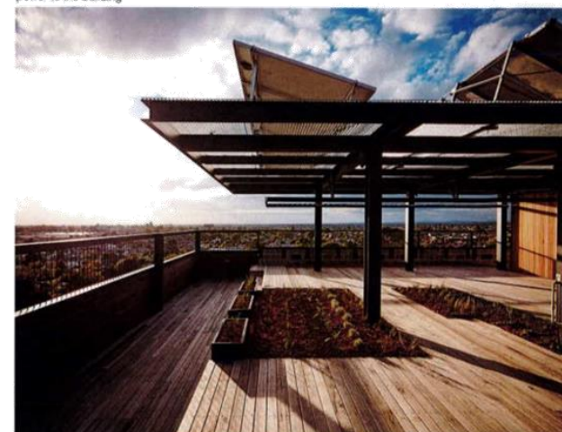
ROOFTOP SOLAR PANELS solar panels are proposed to be located on top of the rooftop terrace sunshade structure to supply base-load power to the building
