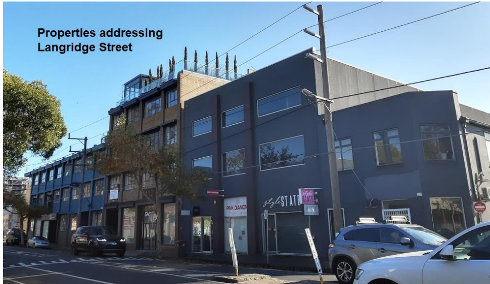
Figure 20: Properties addressed to Langridge Street on the northern side, commencing from the north-west corner of the Rupert Street intersection.
