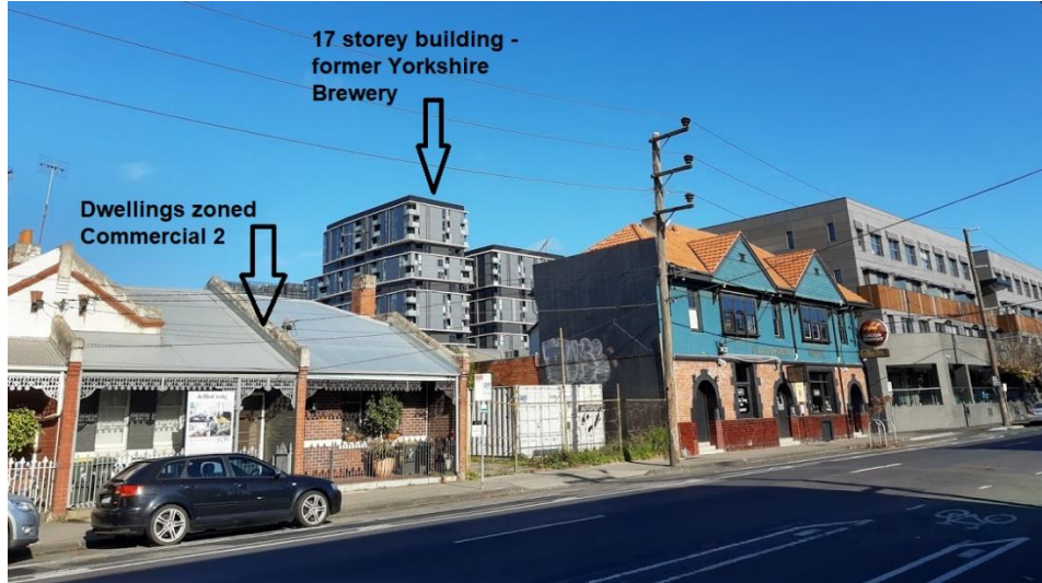
Figure 16: Properties to the south of Gipps Street, between Rokeby and Rupert Streets with the 17-storey, former Yorkshire Brewery in the background.
