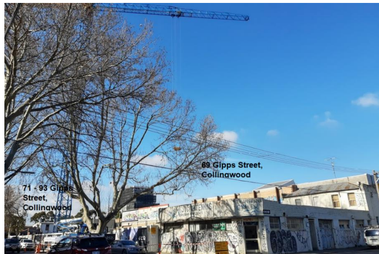
Figure 13: South-east corner of Gipps and Rupert Street, with the land at 71-93 Gipps Street, in the background cleared and cited with a crane in preparation of construction.
