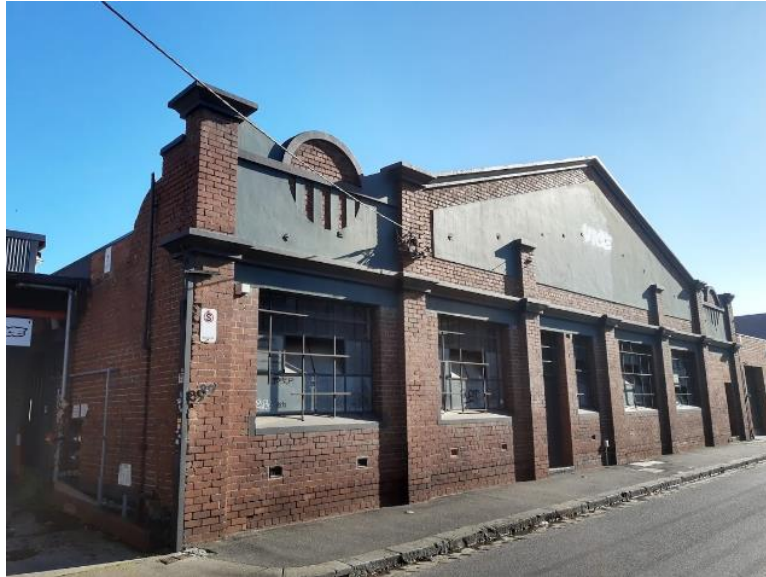
Figure 9: Subject site – Northern portion – former Davis' Pickle and Sauce Factory
