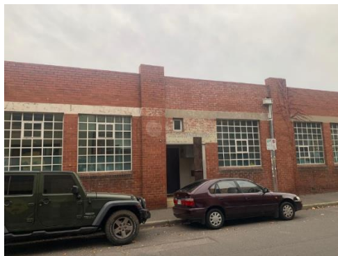
Figure 14: Building directly opposite the subject site fronting Rose and Spring Streets.
