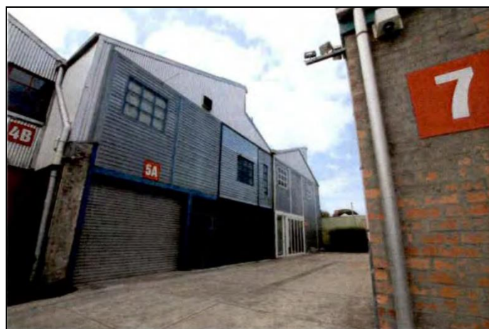
Figure 4 – Nos. 5/1 & 6/1 Bik Lane, Fitzroy North (Source: Applicant)
