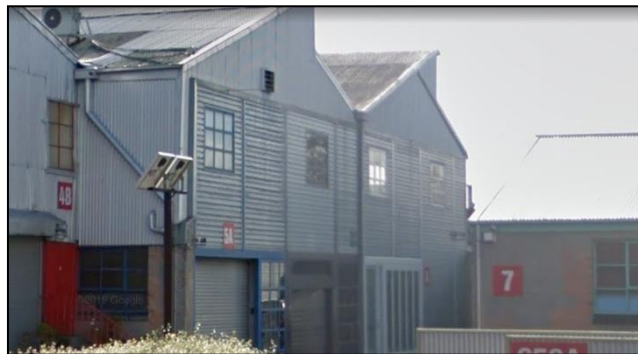
Figure 11 - Southern facades of 5/1 and 6/1 Bik Lane (Source: Google)
