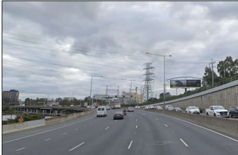
Figure 4 - Existing major promotional signs along the Monash Freeway proximate to the site
