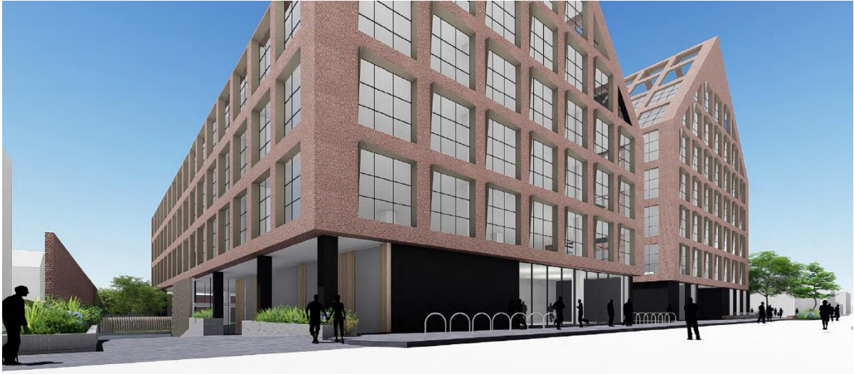
Figure 1: Visualisation of the mixed use development at the subject site which is currently under construction.
