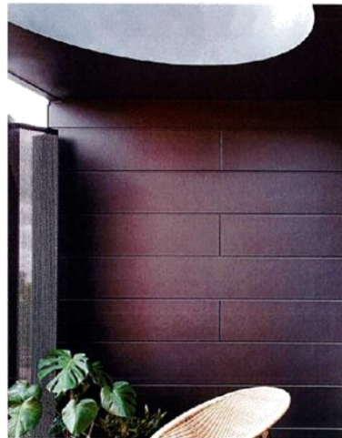
MC-1 METAL CLADDING - DARK Metal Cladding
