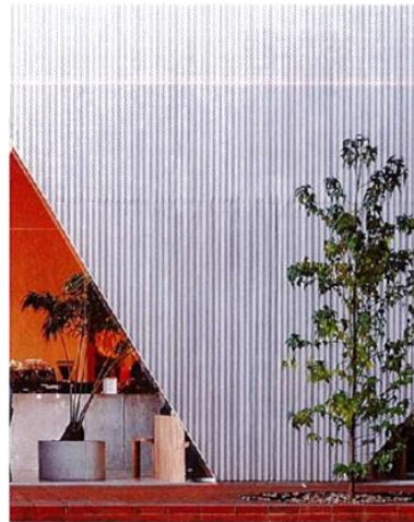
CN-1 CONCRETE Concrete (Formed Profile)
