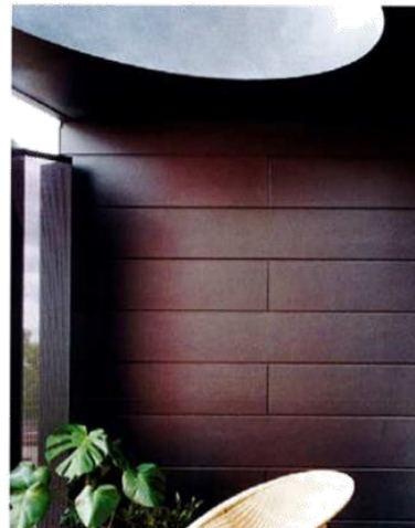
MC-1 METAL CLADDING - DARK Metal Cladding
