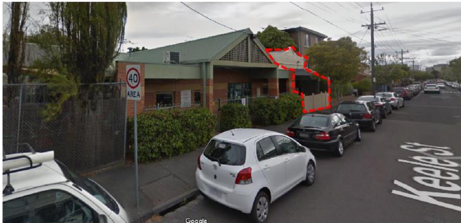
Above: View westwards along Keele Street towards subject site. Subject site denoted by red dashed line.
