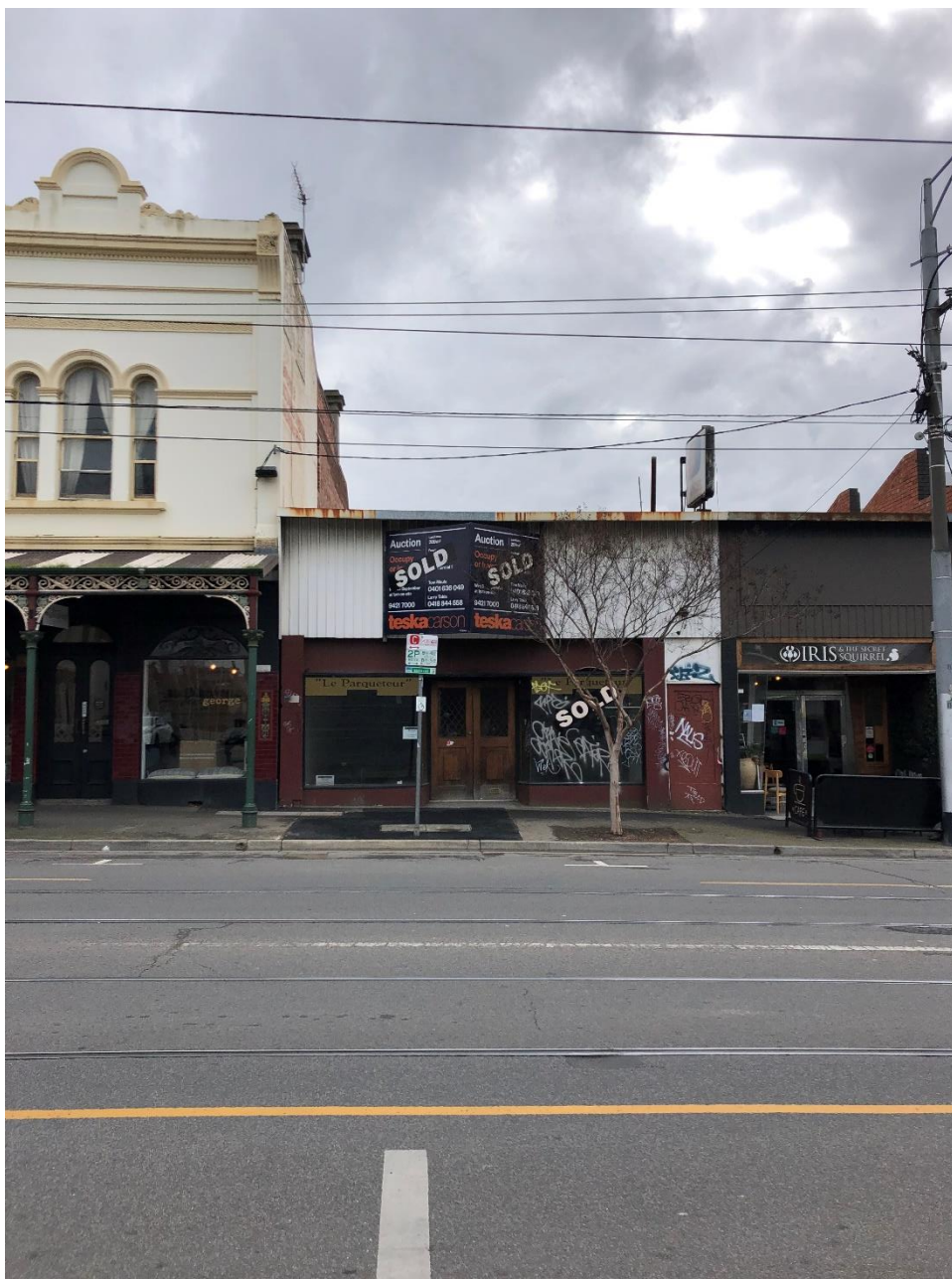
Image 1: Photo of the subject site facing north (taken 14 August 2019)
