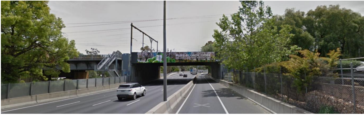
Major promotional sign on railway bridge (electronic)
