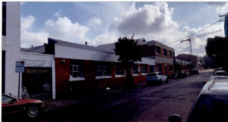
Figure 3 – view of subject site from the looking south-west in Keele Street
