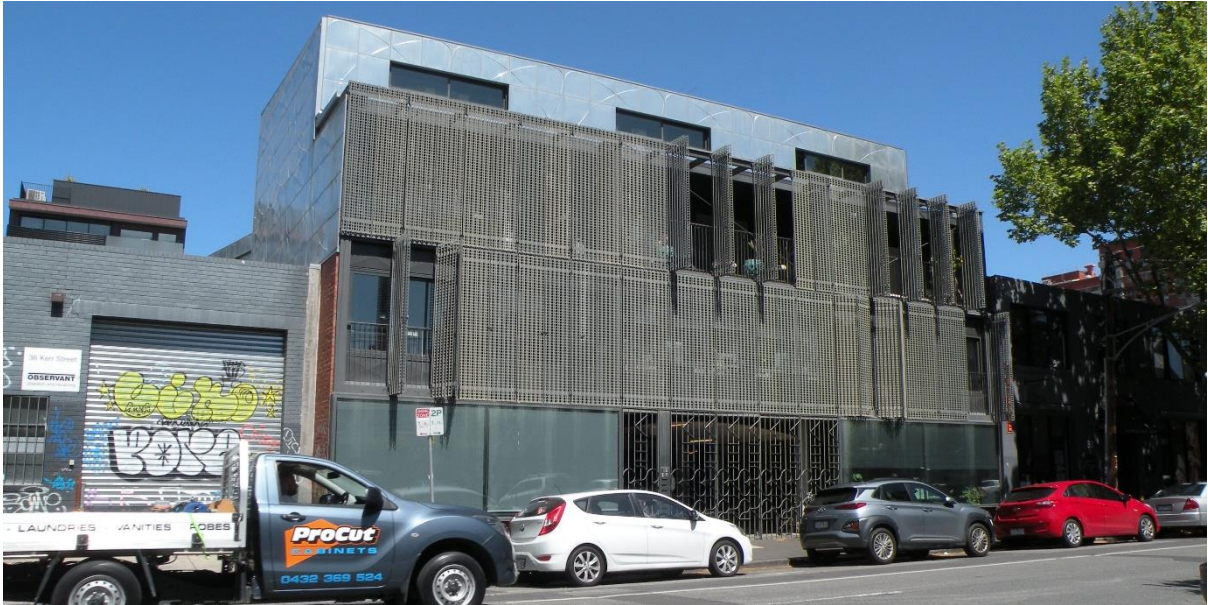
Adjoining building to the west
