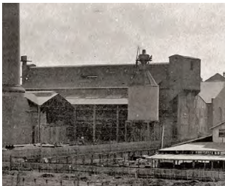
Boiler Room: Historical envelope & structure
