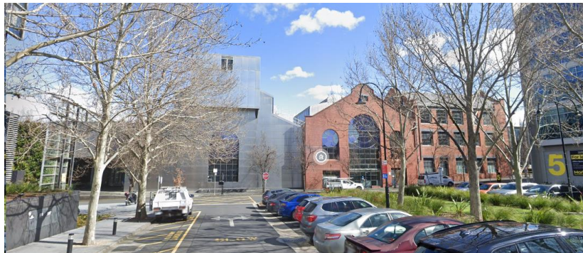
Figure 1. East Elevation (Hargreaves Street), Source: Google Street View 2020.
