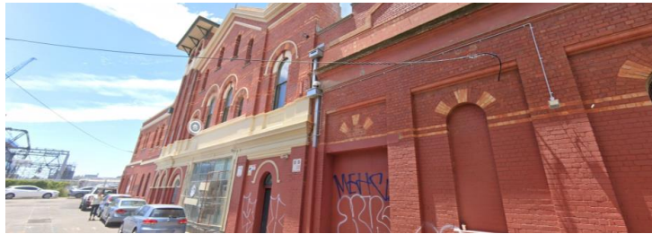
Figure 3. West Elevation (Oddys Lane). Source: Google Street View 2020.
