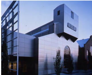
Boiler Room: 90s Facade
