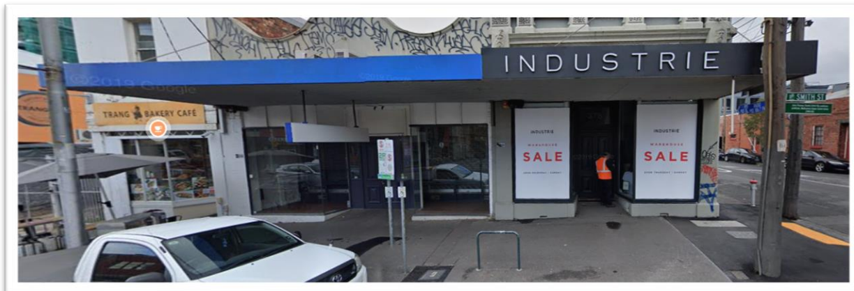
Figure 18- Existing awnings above Smith Street footpath
