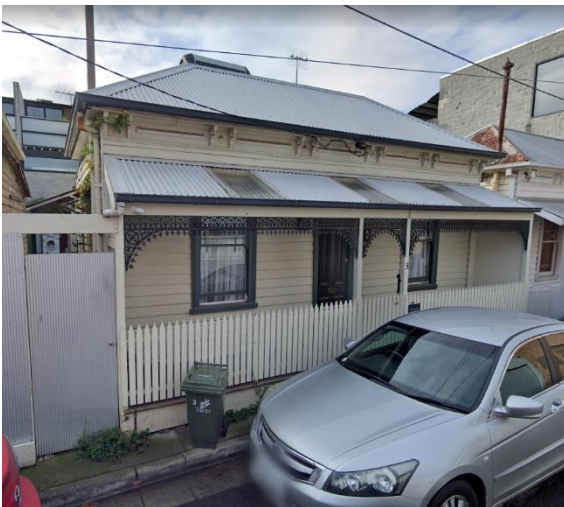
Figure 3: No. 3 Pearson Street, Cremorne (Source: Google Maps, Streetview)
