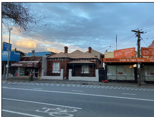
Figure 1 - Subject site No. 121 Burnley Street, Richmond (Burnley Street facade)
