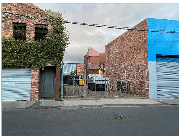
Figure 2 - Subject site No. 121 Burnley Street, Richmond (North Street frontage)
