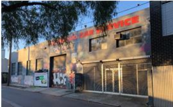
Figure 2: No. 4 – 6 Adolph Street, Cremorne (Source: Officer image, taken 05/07/2019)
