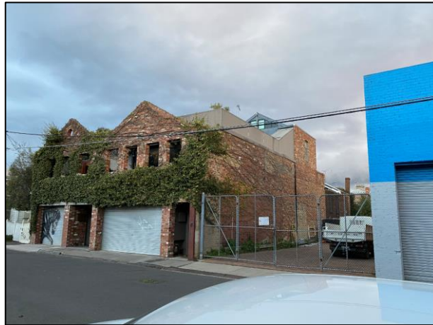
Figure 6 - No. 4 North Street, Richmond - With window constructed along the boundary along third storey visible
