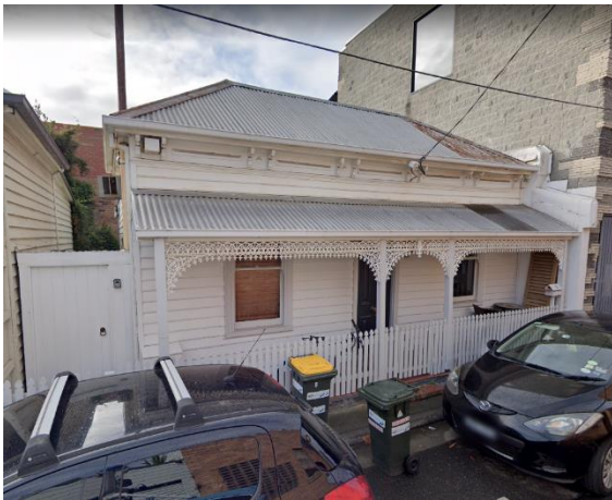
Figure 4: No. 5 Pearson Street, Cremorne (Source: Google Maps, Streetview)
