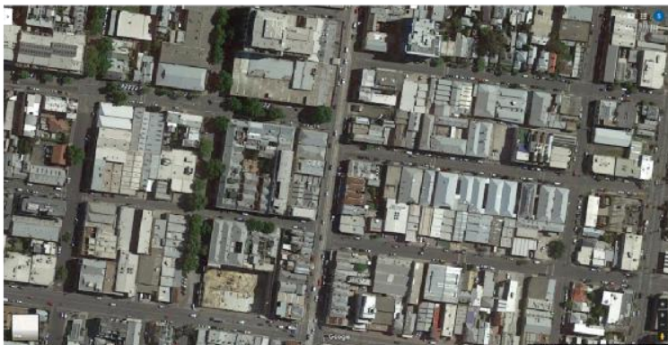
Figure 16: Aerial photograph, Johnston Street to Keele Street, showing predominantly narrow, fine grain built form and subdivision along Smith Street, transitioning to larger lots to the north. Commercial/industrial building forms extend further beyond the Smith Street corridor. (image source: Google).
