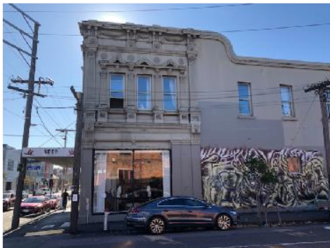
Figure 03: The subject site, Easey Street frontage, at corner of Smith Street.
