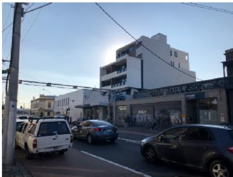
Figure 27: 2 Johnston Street. This narrower contemporary development is approximately 11.5m wide (full site width) with site depth approx. 30.5m and 6 storeys tall. This site at of approx. 350 sq.m is smaller than the subject site.
