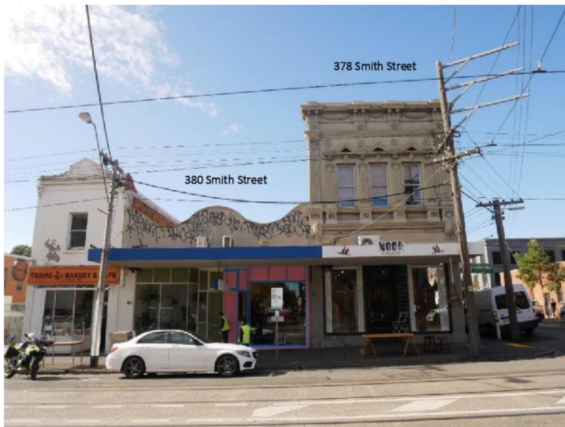
Figure 2. View of subject site from Smith Street, May 2020
