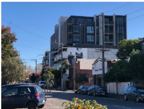
Figure 36: 444-452 Smith Street (7 storeys), Mater Street frontage, looking towards Smith Street, with 3.9m upper level setbacks.
