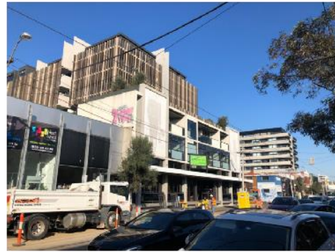
Figure 22: 444-452 Smith Street (looking south-east).
