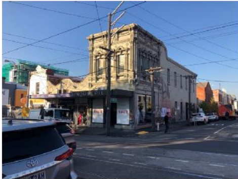
Figure 01: The subject site, viewed from across Smith Street
