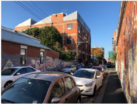
Figure 07: Heritage built form: robust, bold warehouse buildings.
