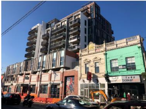
Figure 19: 466-482 Smith Street (looking north-east). This development integrates a heritage street wall element. The upper level tower form reflects a more vertical emphasis through its form and articulation. Built form parameters:
