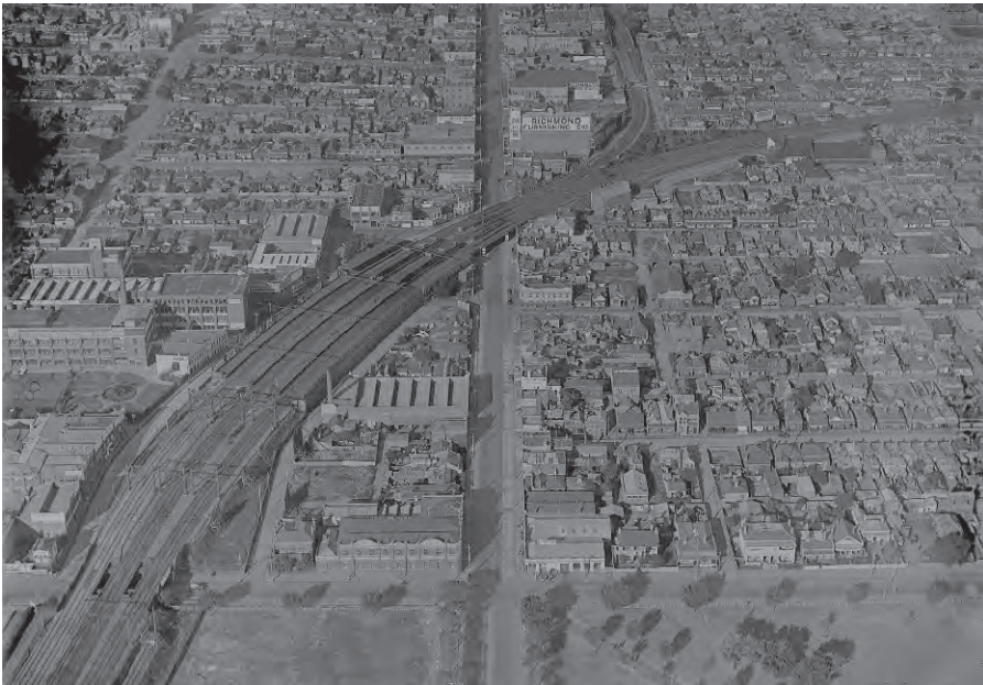
Aerial view of Richmond, between 1924-1939 Source: State Library of Victoria
