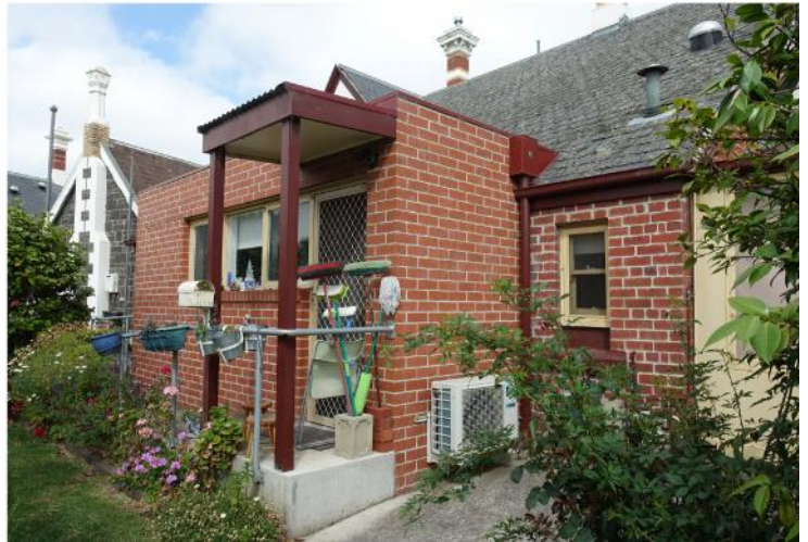
View of south east façade (rear), towards No. 26
