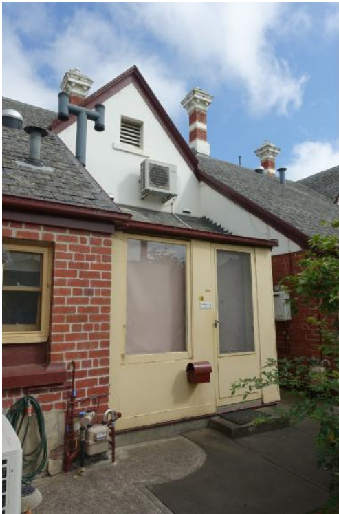
View of south east façade (rear), towards No. 28
