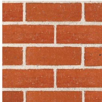
BR1 – Common red face brickwork.
