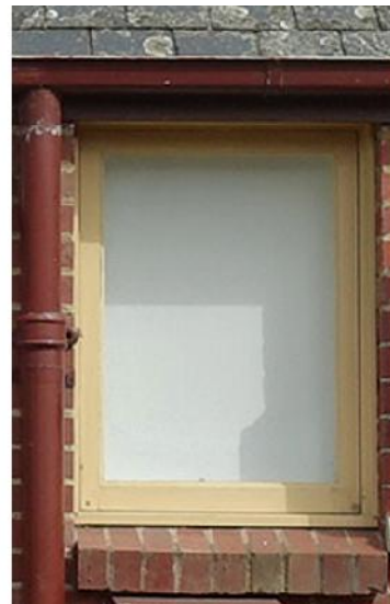
WD – Timber frame windows/doors Paint colour: cream.
