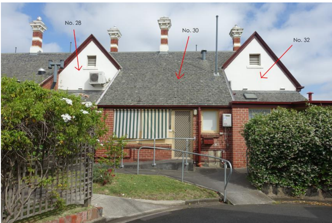
View of south east façade (rear)
