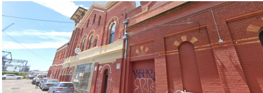
Figure 3. West Elevation (Oddys Lane). Source: Google Street View 2020.
