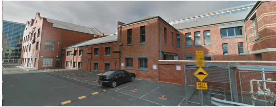
Figure 2. North Elevation (Electric Street). Source: Google Street View 2014.
