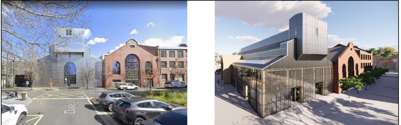
Figure 8: Existing and proposed eastern façade of Boiler House building Source: Design Book (OMA, November 2023)
