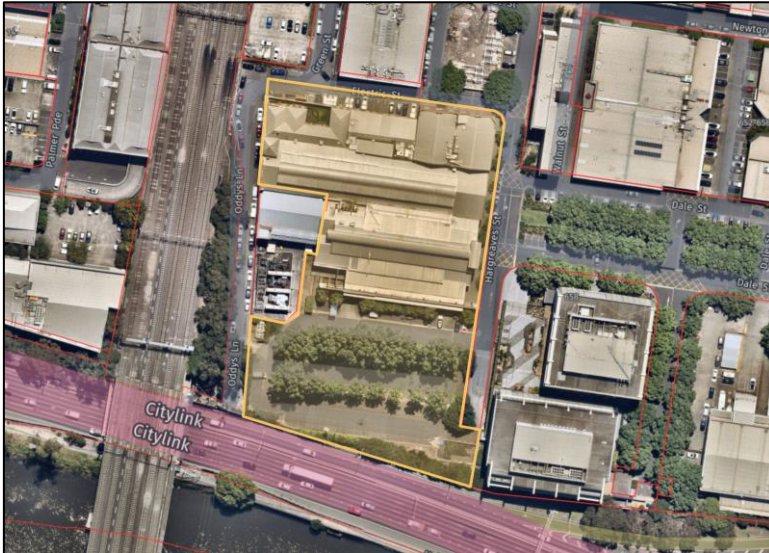
Figure 1: Aerial view showing existing buildings/structures and concrete car parking on-site Source: NearMap, November 2023
