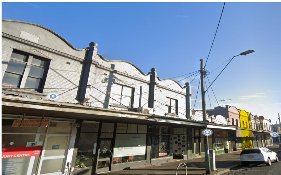
Figure 20: Subject site frontage highlighted in yellow
