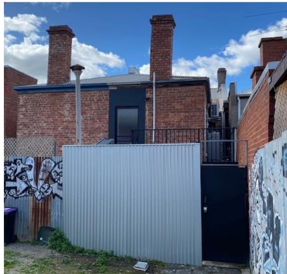
View rear of No's 71 and 73 Smith Street
