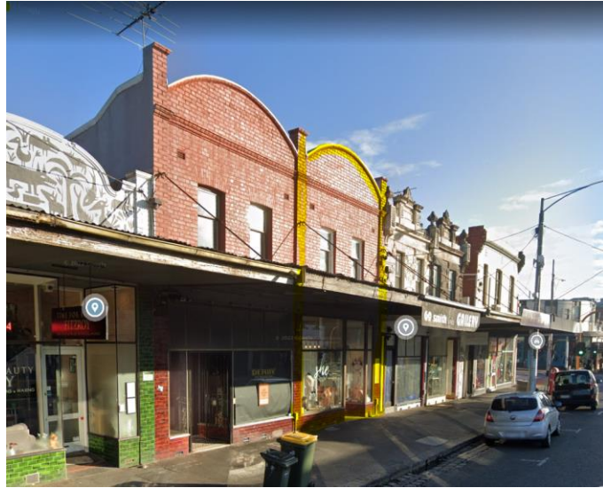
Figure 7: Subject site frontage highlighted in yellow
