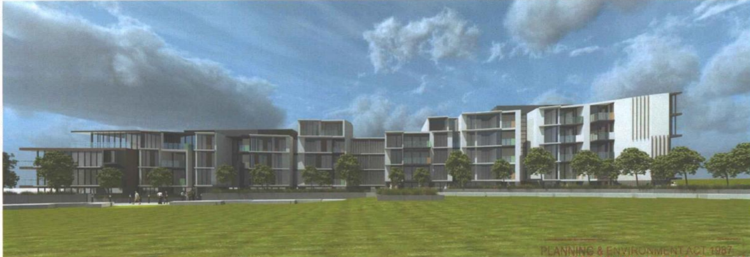
OVERALL VIEW FROM NORTH
