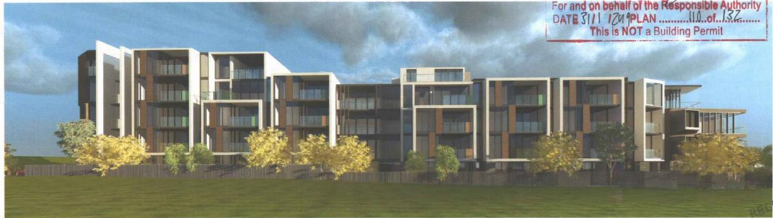
OVERALL VIEW FROM SOUTH
