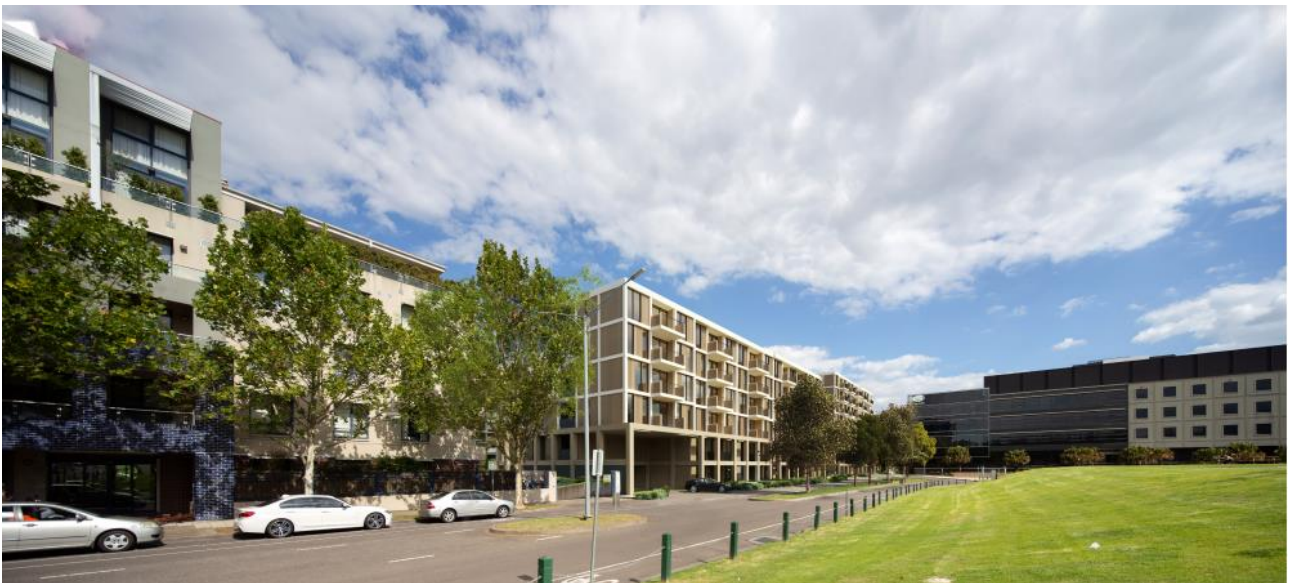
Image: Perspective showing transition of existing and proposed buildings along River Boulevard viewed north of the Site. Source: Urban Context Report, prepared by Bates Smart.
