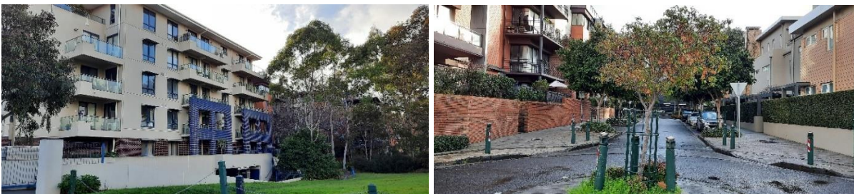
Photos: Existing 5 storey apartment building at 15 River Boulevard viewed from River Boulevard (left) and 10 Elaine Court and 6 Christine Crescent viewed from Christine Crescent court bowl (right)
