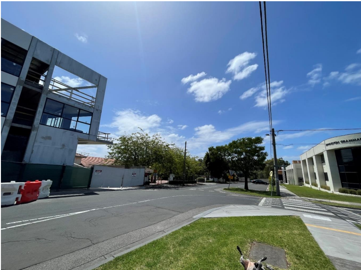
Image 7: Old Heidelberg Road looking east, Alphington Grammar on corner to Lucerne Crescent to the right and the proposed apartments at No. 838 – 852 Heidelberg Road to the left (Officer site visit, January 2023)
