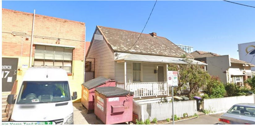
Figure 10: Property No's. 17 – 19 (extracted from Google – Image capture Nov. 2021)
