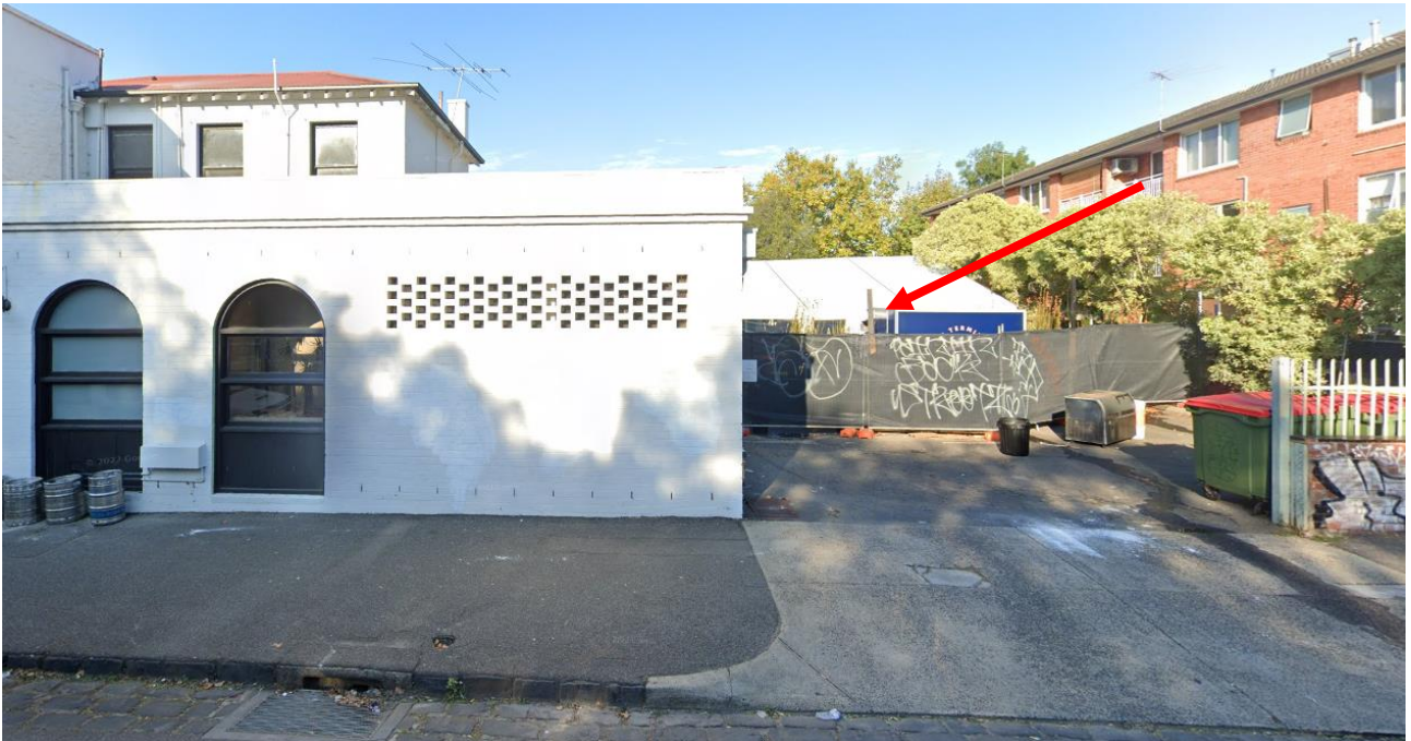
Figure 2: View of Brennand Street frontage and approximate location of new rear addition red arrow (source: Google StreetView)
