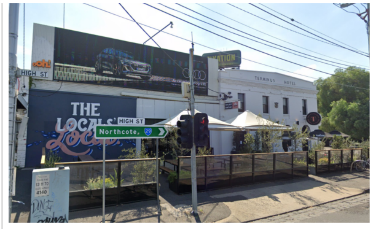
Figure 2: Building façade addressing Queens Parade
