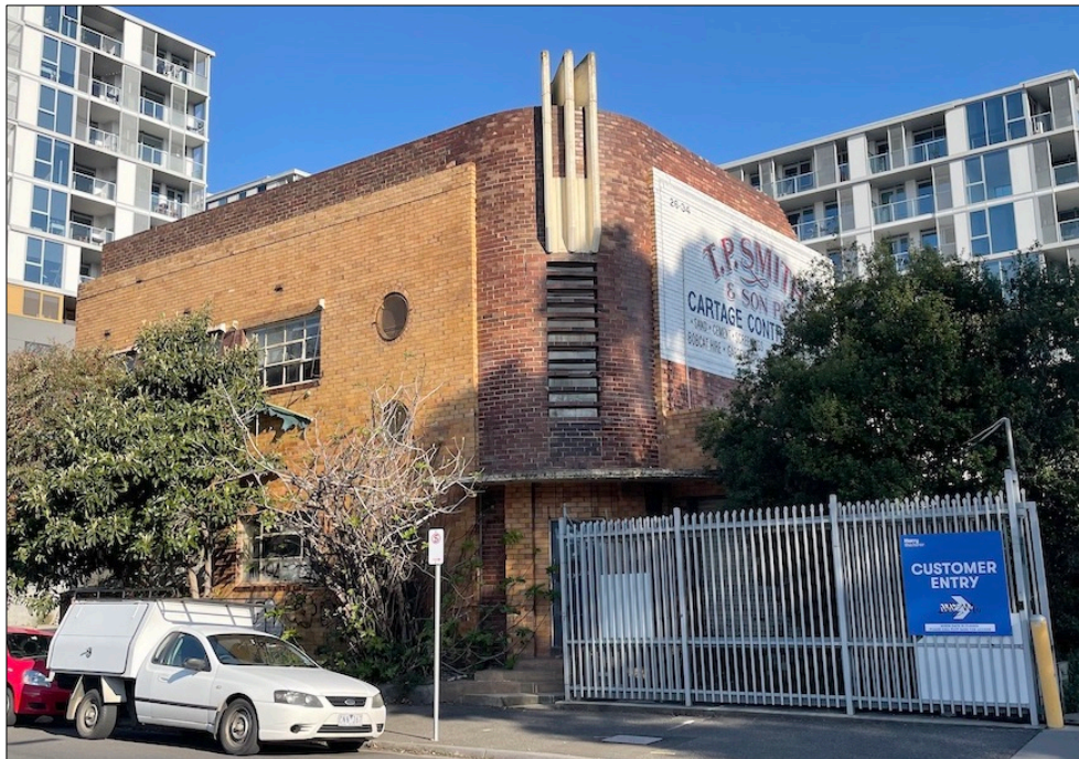
Figure 13 The former Repco building at 26 Doonside Street, located at the eastern end of the subject site.
