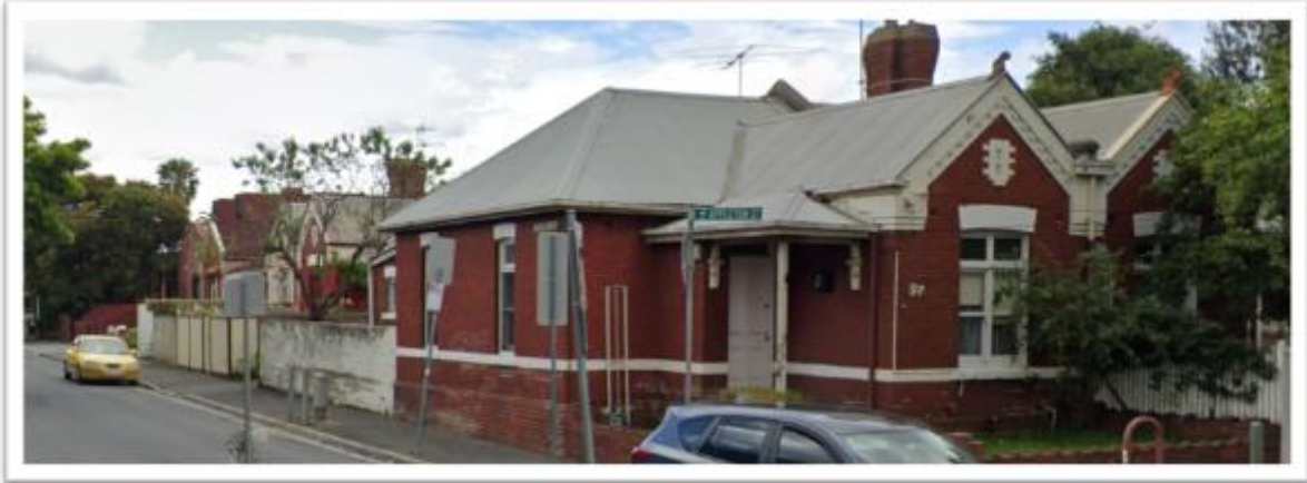
Figure 19: View along Appleton Street
