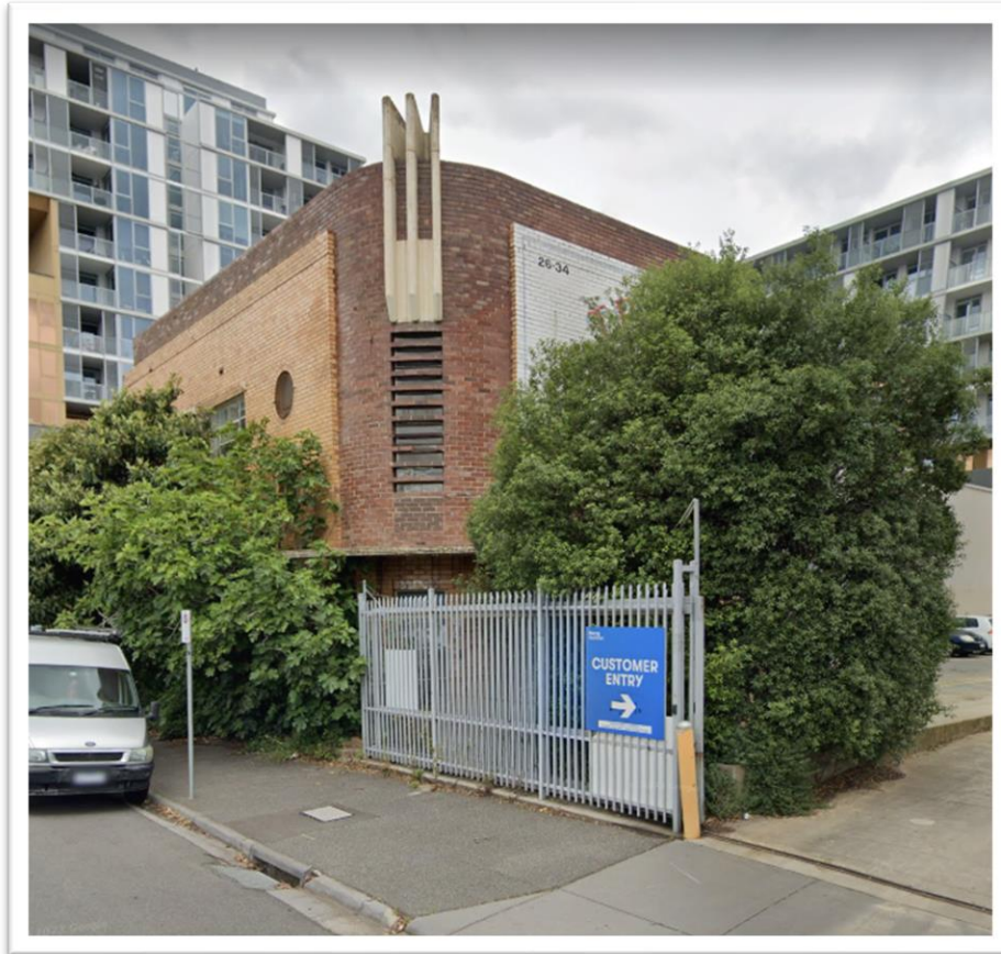
Figure 10: former Repco Offices and Laboratories (26 Doonside Street). Source: Landscape Plan (TCL 2023)
