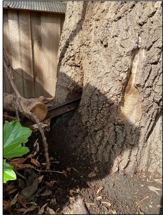
Tree #1, the stem base. A cavity (the steel picket was taken out to inspect the cavity) and a minor wound.
