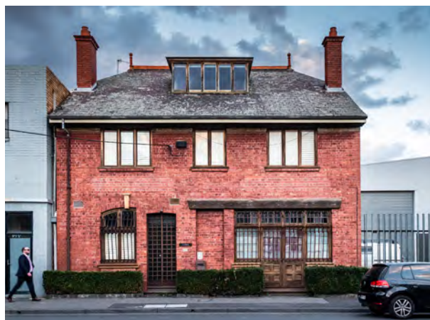
Image 76 - Former Yarra Hotel Cremorne Street
