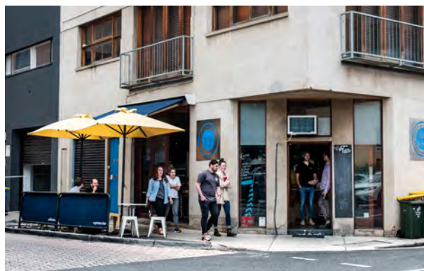
Image 50 - Chamfered building corners
