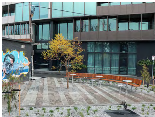
Image 18 - Recent Gwynne Street upgrades
