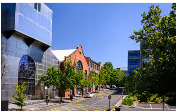
Image 71 - 658 Church Street - Former Power Station
