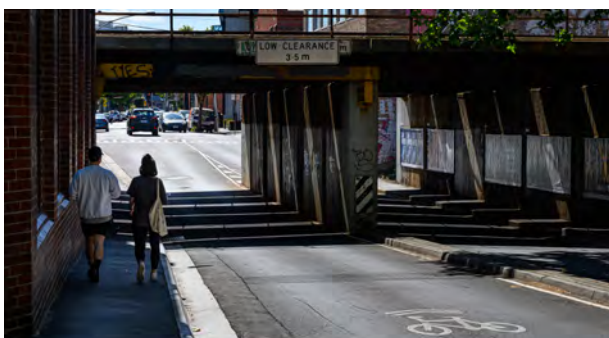
Image 22 - Balmain Street underpass
