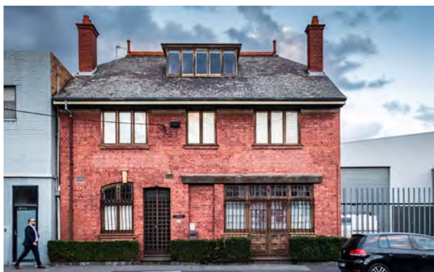
Image 67 - Former Yarra Hotel Cremorne Street
