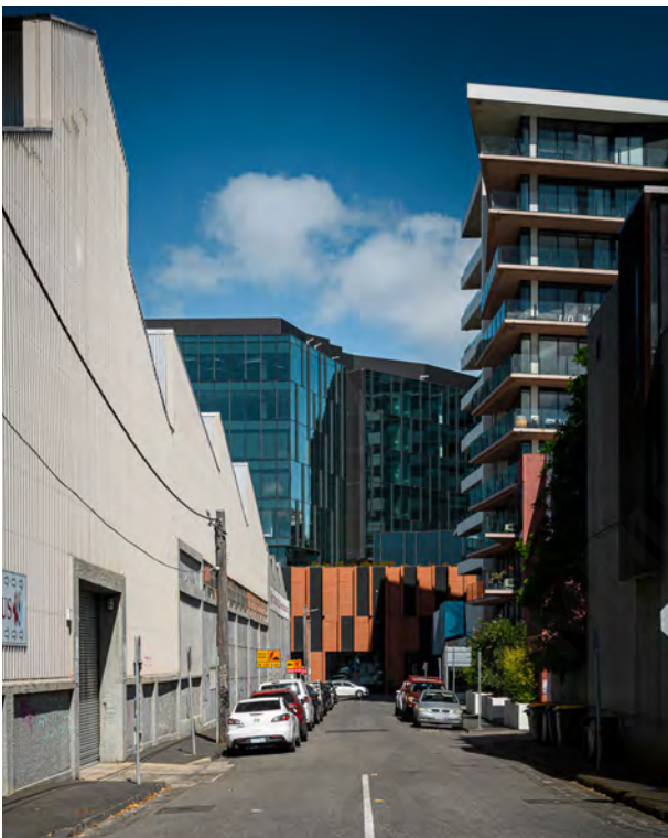
Image 83 - Bent Street existing warehouse
