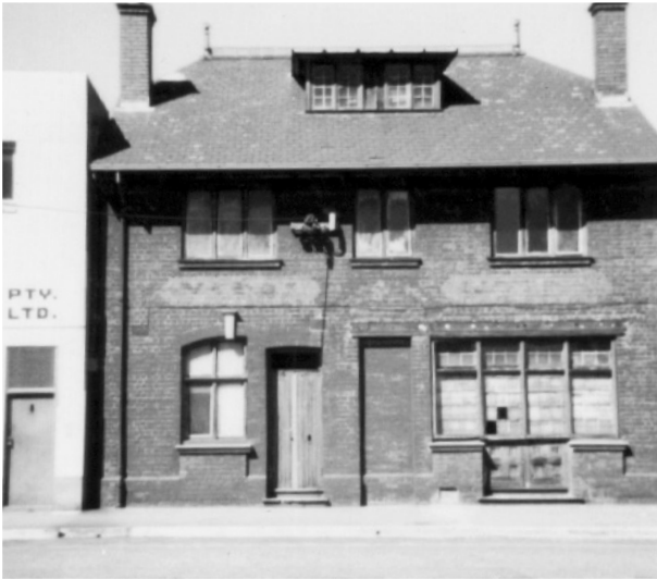
Image 5 - Former Yarra Hotel (Cremorne Street)
