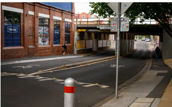
Image 25 - Balmain Street rail underpass
