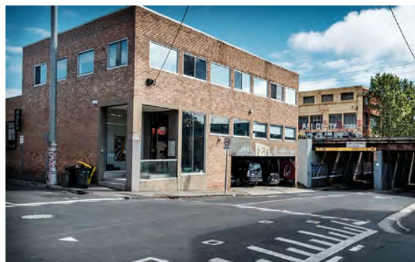
Image 77 - Balmain Street underpass looking west
