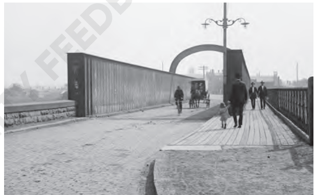
Image 4 - Church Street bridge (1914)
