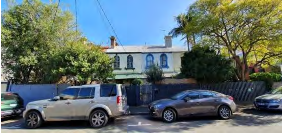
Figure 33. 30-38 Dover Street. Source: Trethowan Architecture.
