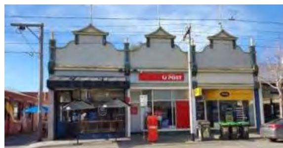
Figure 40. 533-537 Church Street. Source: Trethowan Architecture.
