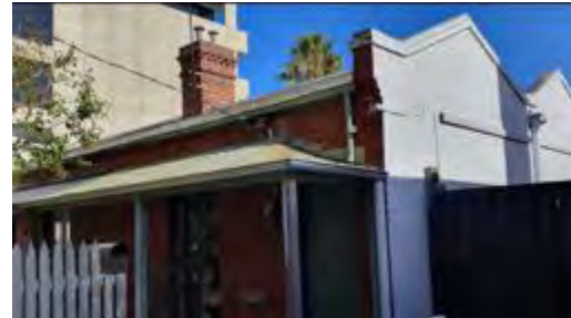
Figure 30. Detail view of the side gables. Source: Trethowan Architecture.
