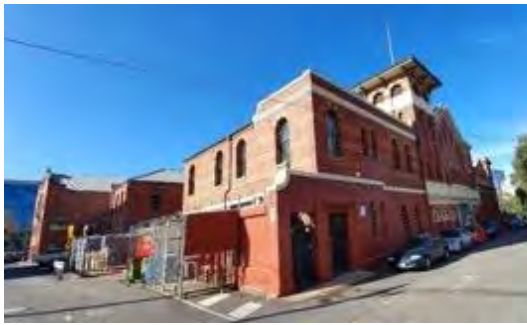
Figure 46. North-western elevation with tower. Source: Trethowan Architecture.
