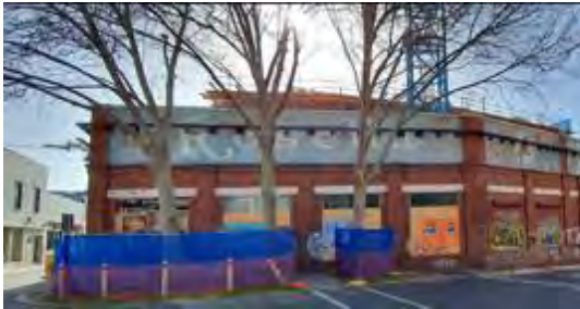
Figure 52. Current development site north of Balmain Street, Building 1. Source: Trethowan Architecture.
