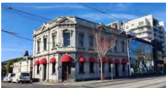
Figure 39. 619 Church Street. Source: Trethowan Architecture.
