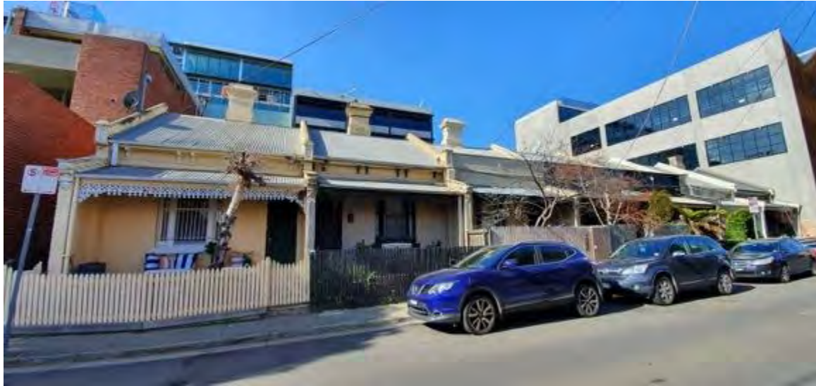
Figure 31. The terrace at 21-33 Cubitt Street. Note sheer wall elevation on the south. Source: Trethowan Architecture.
