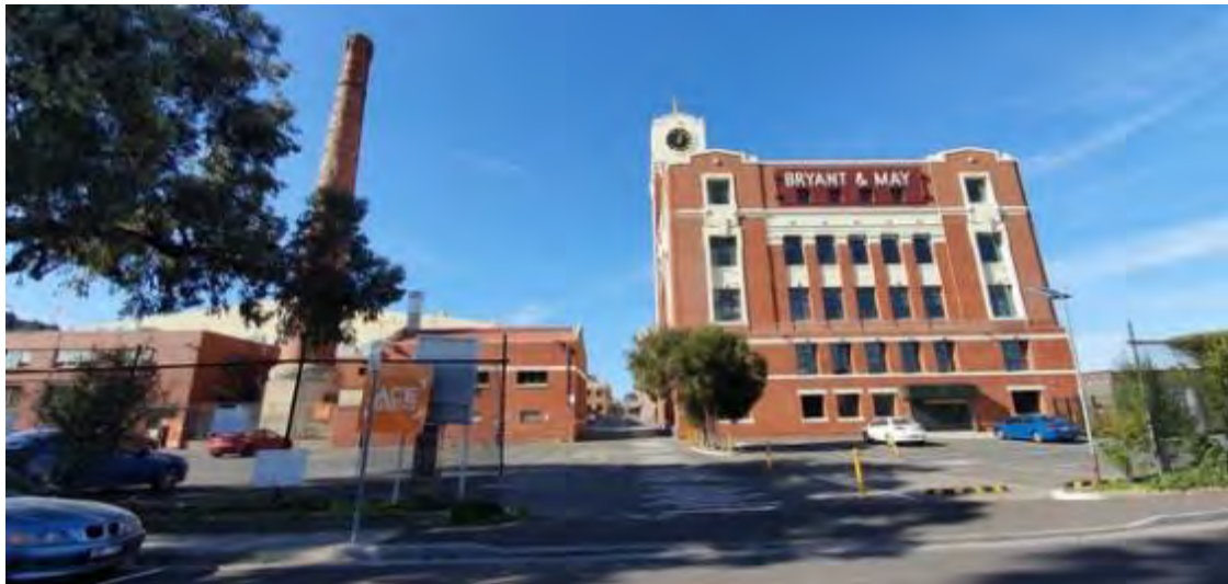
Figure 42. View through the Bryant and May site from the immediate west. Source: Trethowan Architecture.
