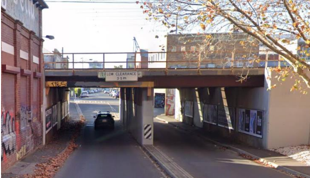
Figure 4.6 – Existing Balmain Street Underpass
