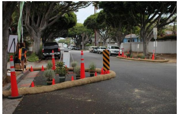
Figure 4.4 – Pinch point trial on a local street using sandbags to create the kerb build-out
