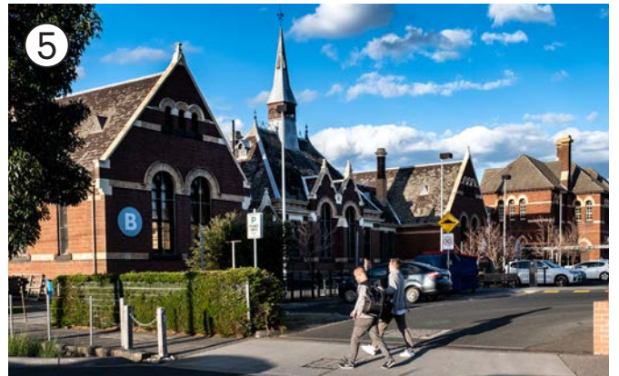
Image 26. Former Richmond Primary School as viewed from Cremorne Street.
