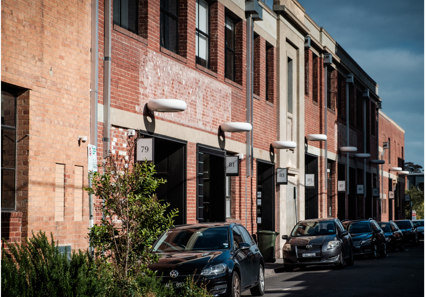
Image 1. Typical industrial buildings found in Cremorne.
