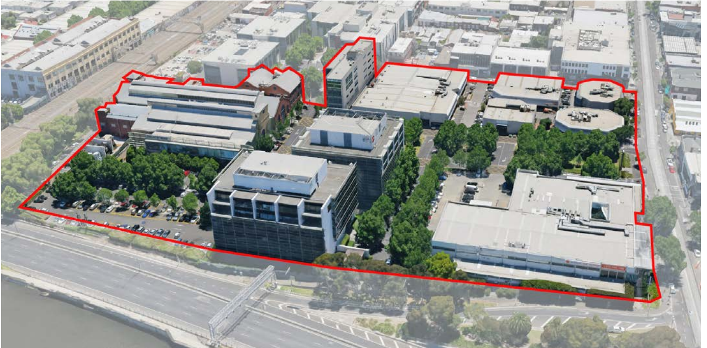
Figure 90. 658 Church Street aerial
