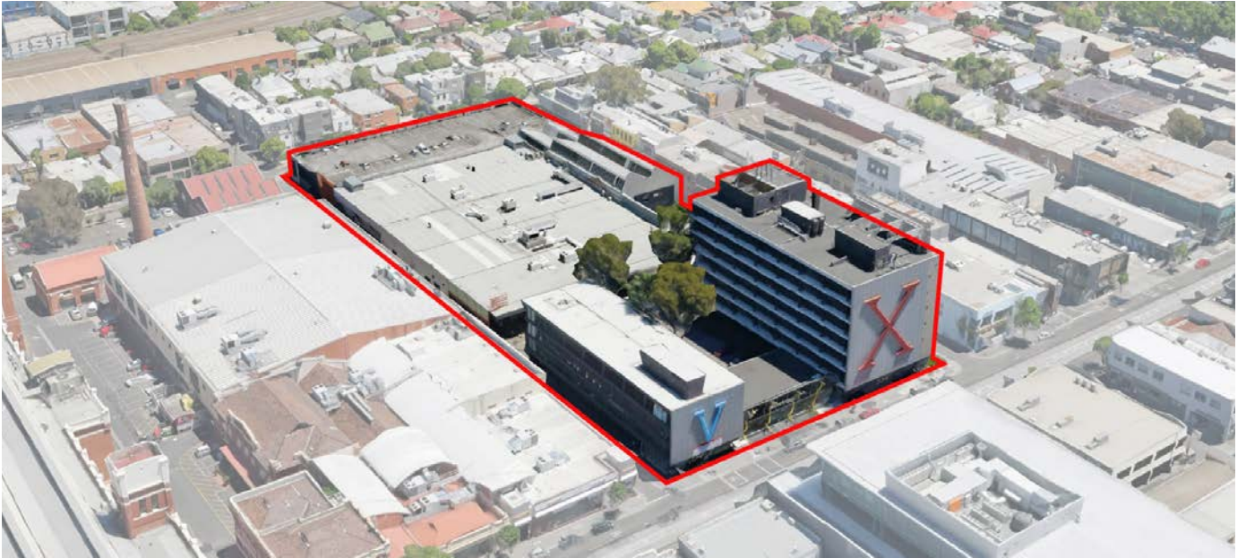
Figure 84. 534 Church Street aerial
