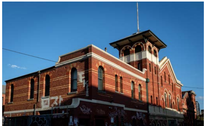
Image 9. A view of the Richmond Power Station on Green Street.
