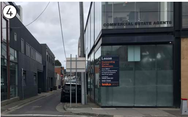
Image 19. Poor example of ground floor design on Church Street with floor to ceiling glazing and limited architectural detailing.
