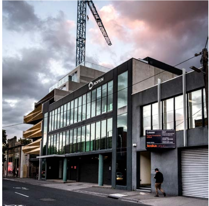
Figure 30. Buildings of between 2 and 6 storeys along Cremorne Street.
