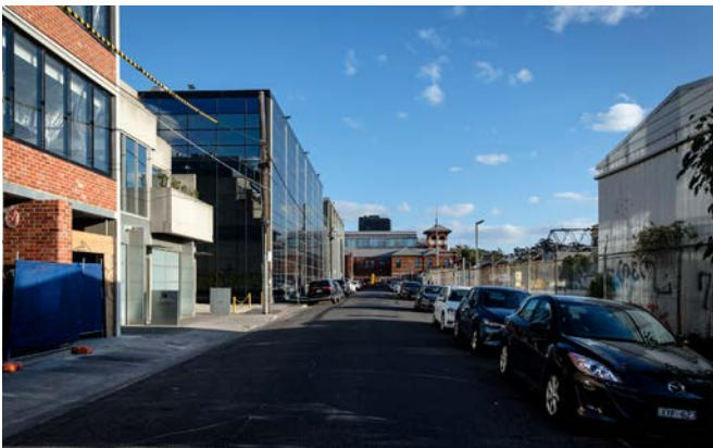
Image 38. Looking south along Green Street towards Richmond Power Station.
