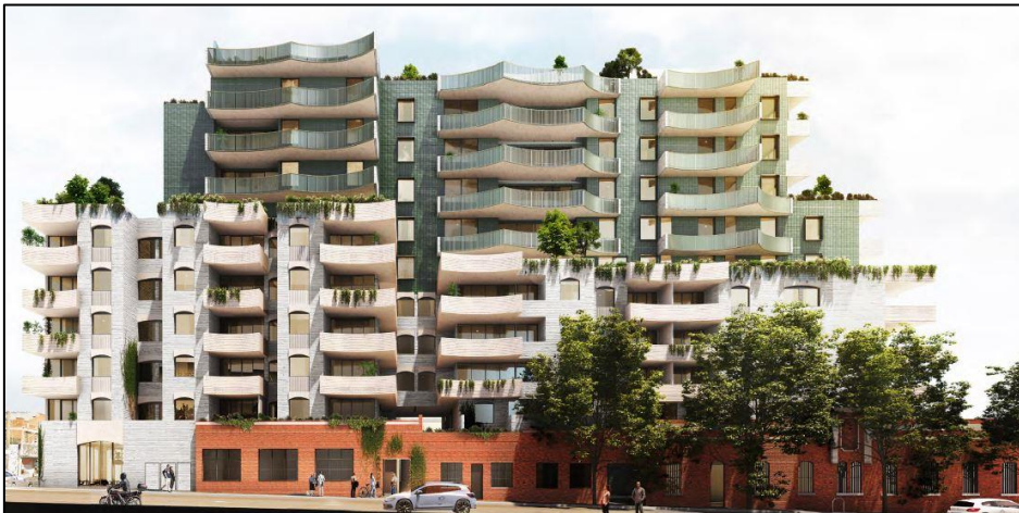
Figure 38: Previous - Gore Street Façade (SJB Architects March 2020)
