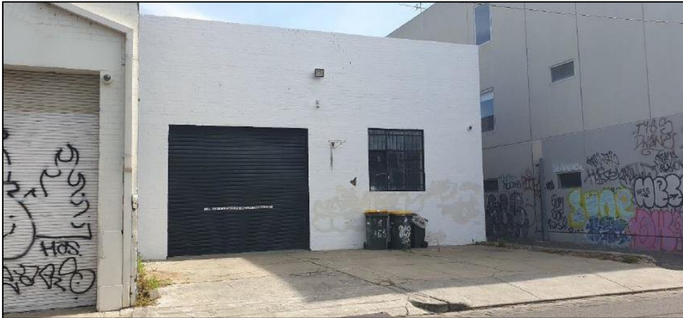
Figure 22: Subject site – Argyle Street façade (Urbis, November 2021)
