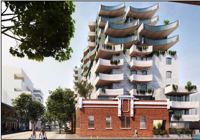
Figure 40: Previous - Argyle Street Façade (SJB Architects September 2021)
