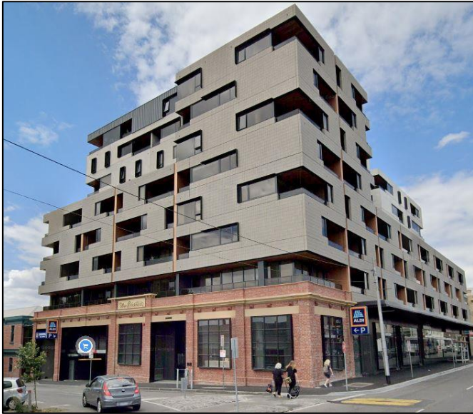
Figure 27: Nos. 239 – 249 Johnston Street (Google Street View, January 2021)
