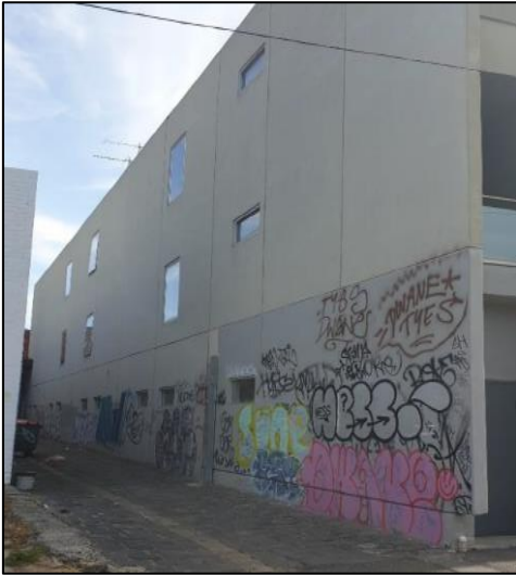
Figure 29: Eastern boundary wall of No. 192 Argyle Street (Urbis, November 2021)
