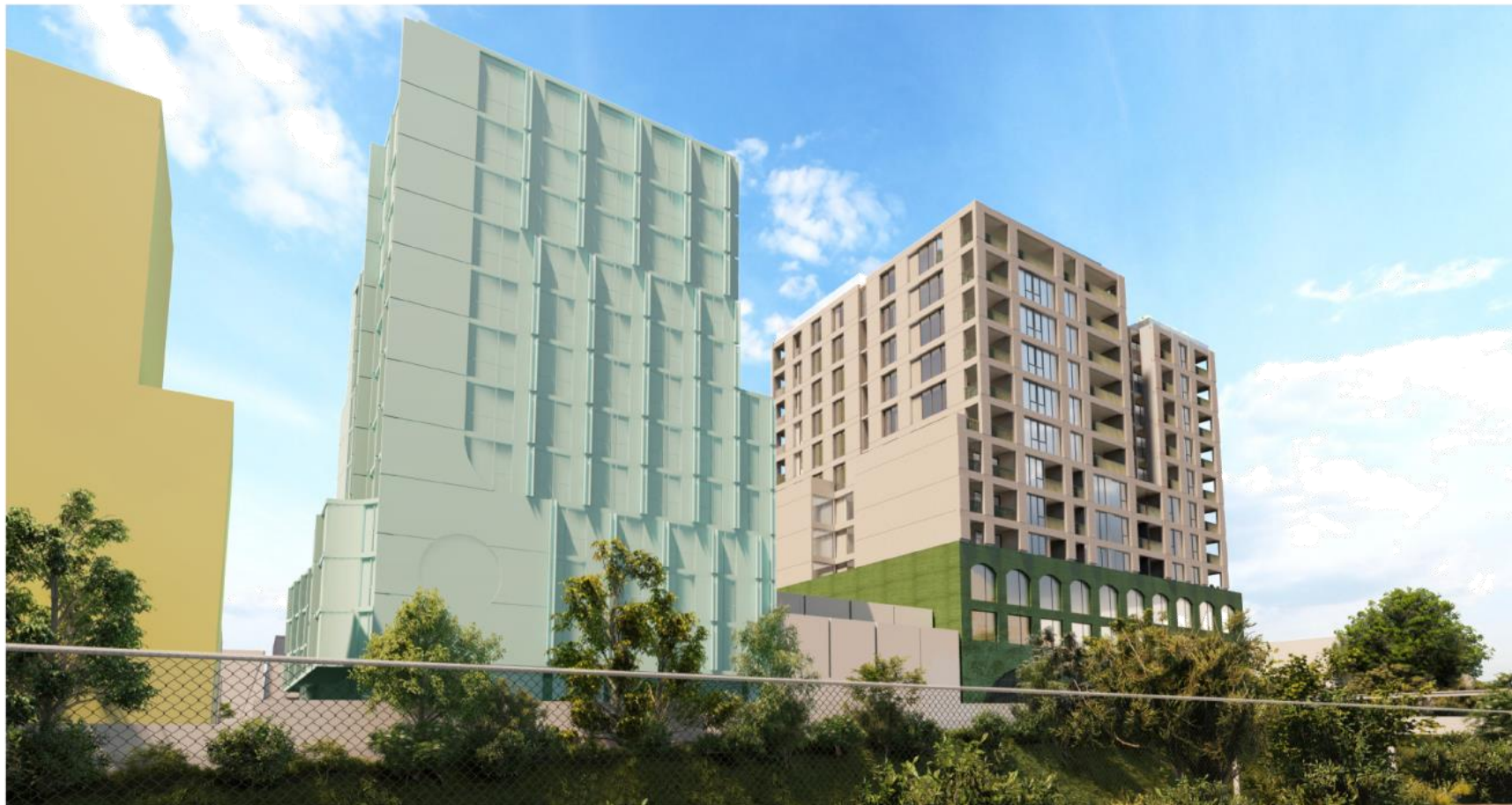
1.7 RFI Item 5A - View from Lesney Street Looking North-East
