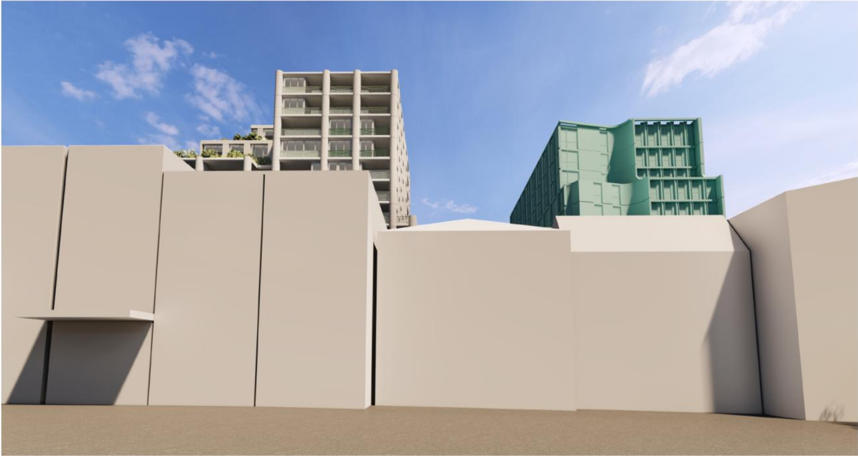
3.23 RFI Item 5D i - View in Front of 205 Swan Street
