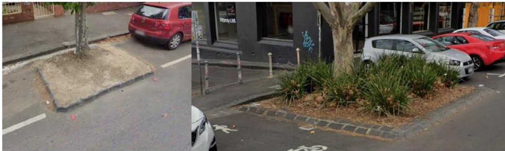
Figure 2: Vehicular outstands to established trees on Gore Street and Westgarth Street, Fitzroy.
