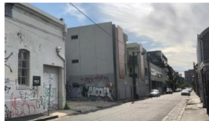
West – 3 storey residential building at 192 Argyle Street
