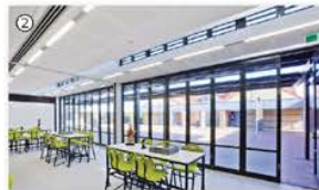
Indoor spaces designed for enhanced air quality, noise control, daylighting, and glare mitigation
