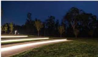
Public Lighting - Providing an integrated lighting approach to the public interface
