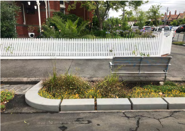
New garden bed in the road space includes slotted kerbing to help capture runoff.
