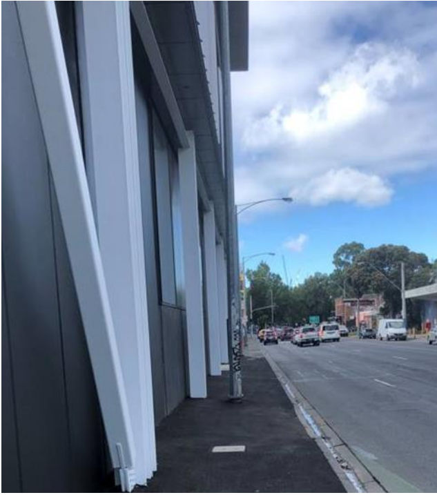
Figure 11 - George Street looking South adjacent to the Wurun Senior Campus
