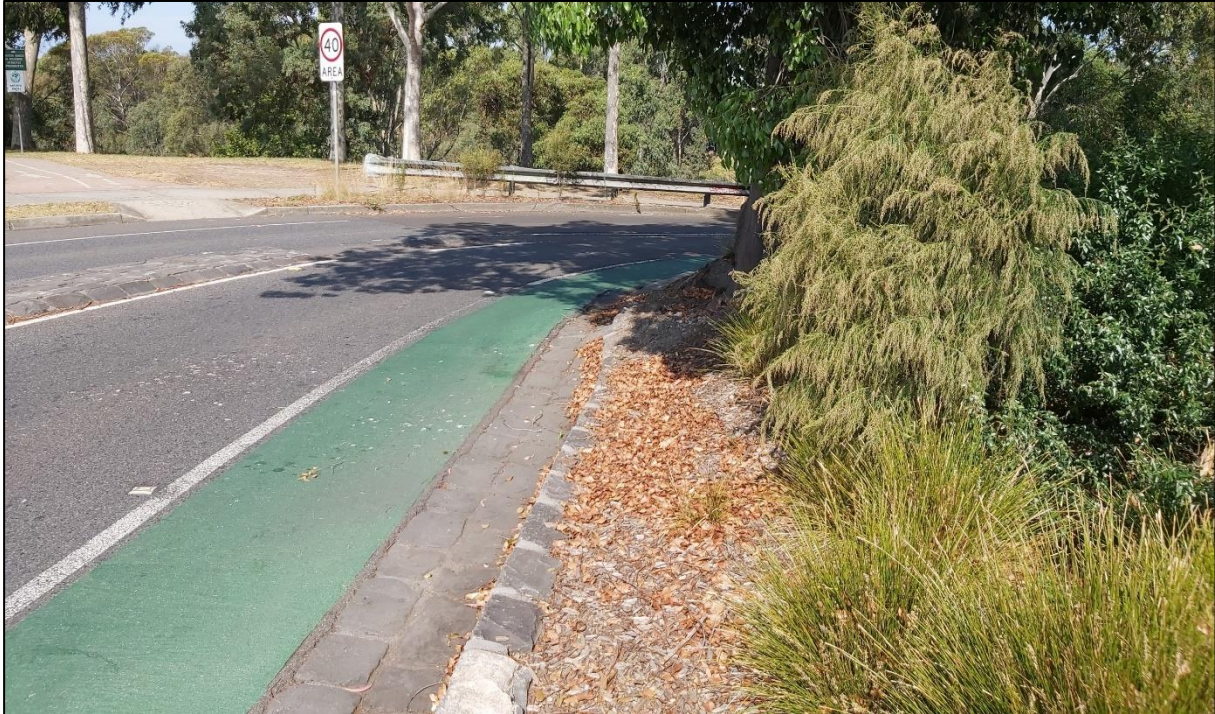
Figure 22: Noone Street / Gray Street / Trenerry Crescent - Poor Pedestrian Crossing Sight Distance
