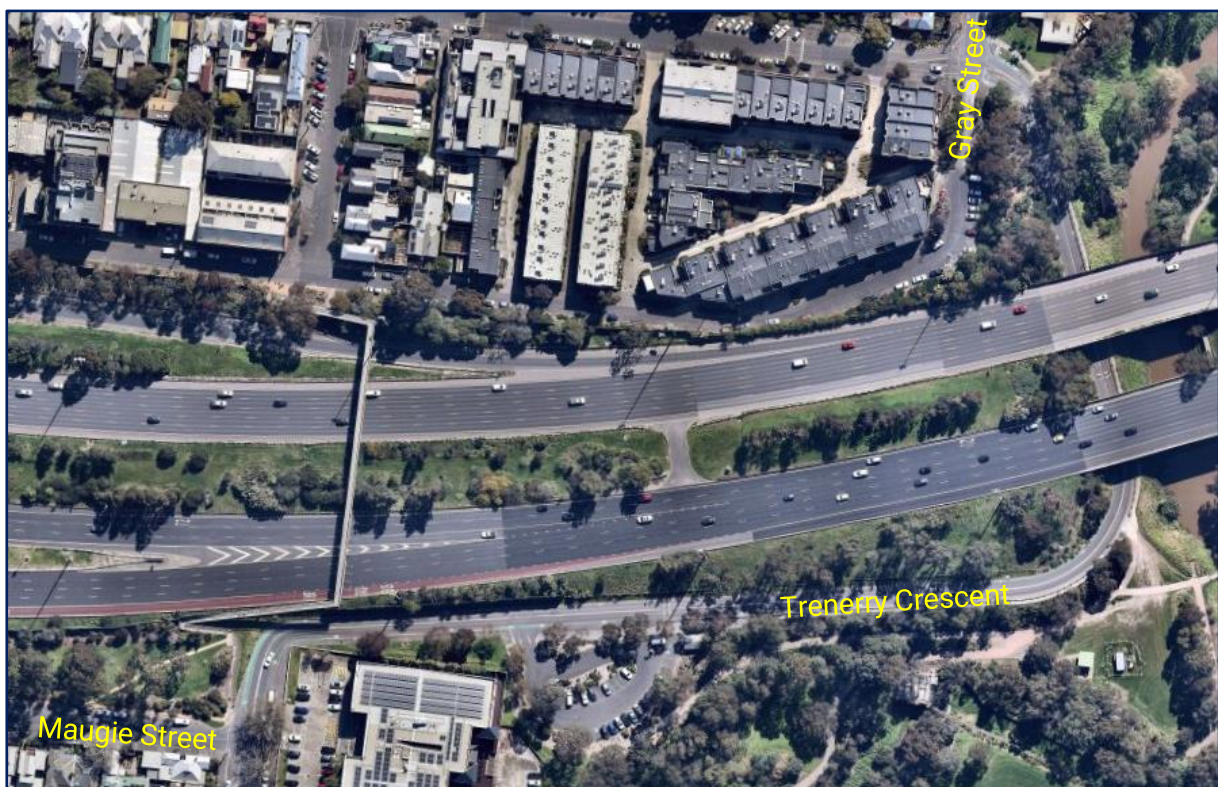
Figure 23: Trenerry Crescent between Gray Street and Maugie Street - Aerial Photograph
