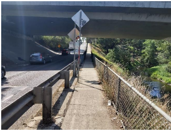
Figure 24: Trenerry Crescent Underpass - View North
