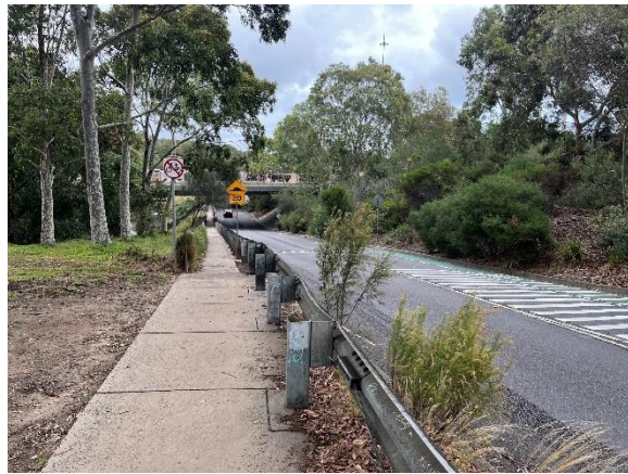
Figure 25: Trenerry Crescent Underpass - View South
